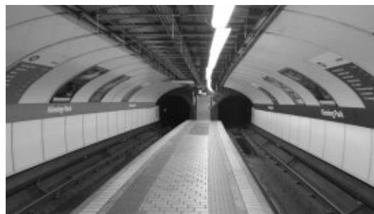
Abb. 2: Station Kinning Park der U-Bahn Glasgow
